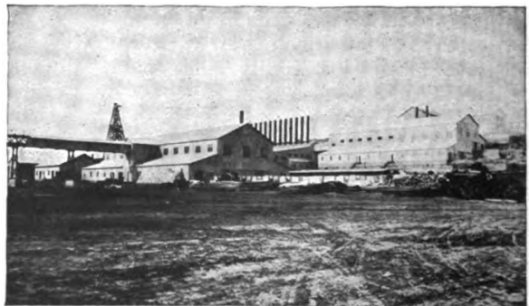
WHERE PORTLAND CEMENT IS TURNED OUT AT THE RATE OF 5,000 BARRELS A DAY
